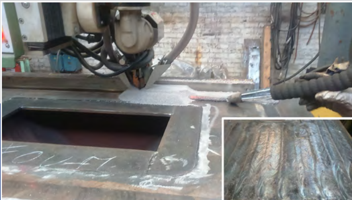
Strip cladding process
